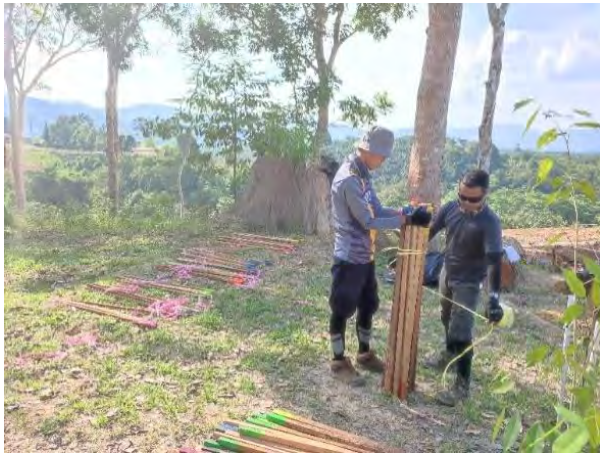
Figure 15. Coloured wooden poles were used to mark the planting holes.
